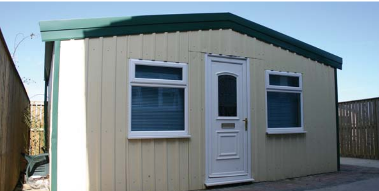
02 Utility Buildings used as office accomodation etc.
