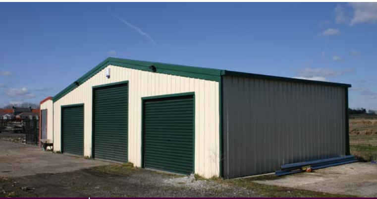
01 Triple Garage with low profile wall cladding
